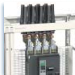
Upstream connection by cables
